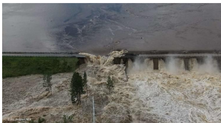
Figure 4: Overtopping of the embankment at dam Braskereidfoss (Photo: Politiet/NVE)
