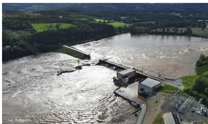
Figure 3: Dam Braskereidfoss during the embankment dam failure (Photo: Police/NVE)
