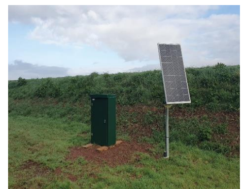
Figure 3: A completed PRIME system installation at Powderham Banks. All cables are buried for protection and to minimise visual intrusion. The system is fully autonomous and operates on solar power.
