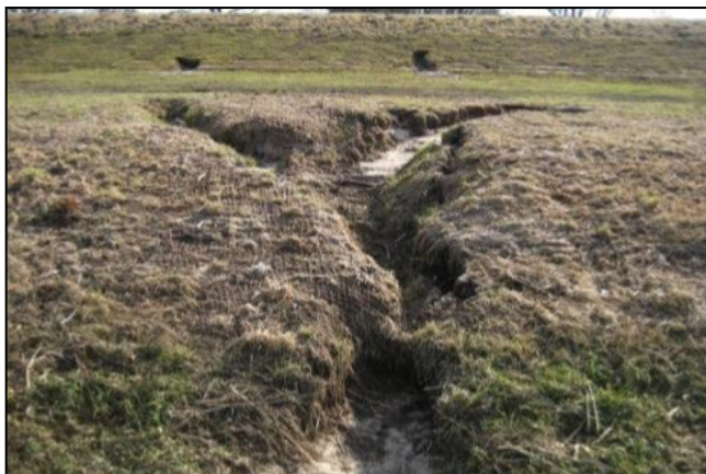
Figure 2: collapsed beaver tunnels, embankment Odra river, in the background: new entrances inside the dyke line (Source: LFU Brandenburg)
