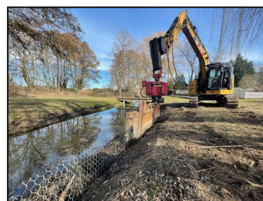
Figure 4 & 5: Barrier installation and detail of the 3-layer compound - netting between two sheet pile plates, embankment section Brandenburg area Biegen, Germany, barrier depth 3,0m (Source: SECON)
