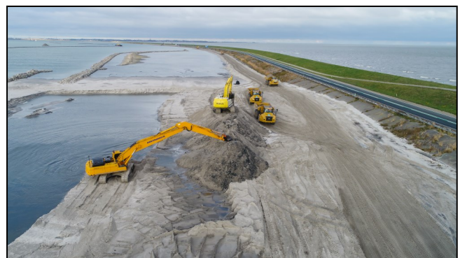
Figure 12: Levee reinforcement with the aid of a new foreshore, located along parts of the Houtribdijk, a levee-like dam separating Lake IJssel and Lake Marken, and connecting the towns of Enkhuizen and Lelystad (Photo by Rijkswaterstaat)
