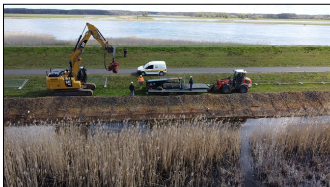
Figure 6: Excavator with vibration device, hydraulic working platform, dyke section along Odra River area Gross Neuendorf, Germany, barrier depth 4,5m (Source: IWT)
