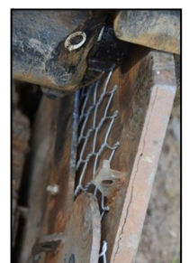
Figure 4 & 5: Barrier installation and detail of the 3-layer compound - netting between two sheet pile plates, embankment section Brandenburg area Biegen, Germany, barrier depth 3,0m (Source: SECON)
