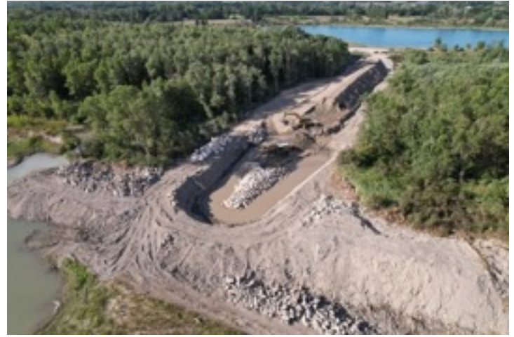
Works to set back and lower the groynes of the Carriers dyke
