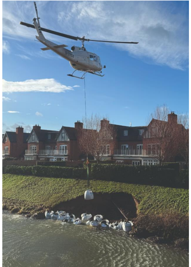
Figure 1: Helicopter helped to fill the Taplow scour area with rock bags
