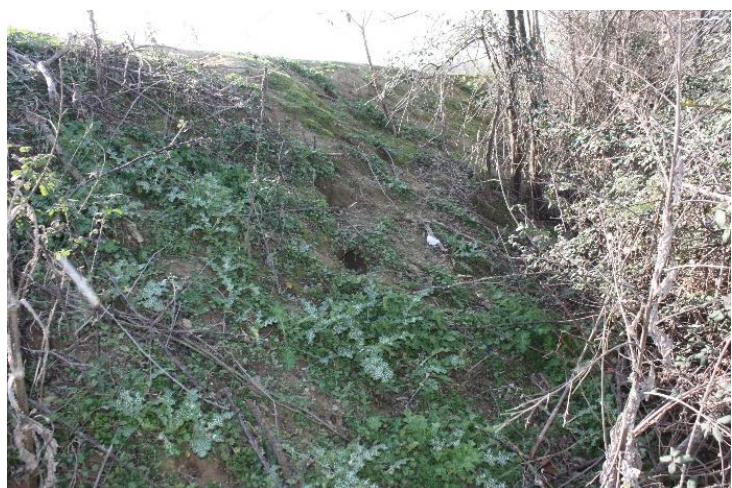
Figure 5: Rabbit burrows on the untreated embankment, February 2020 (photos S. Nicaise)
