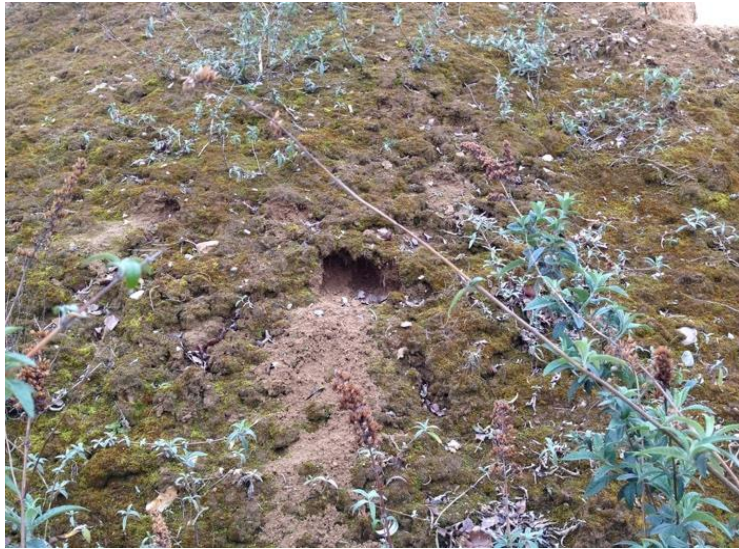
Figure 2: Rabbit holes dug into the untreated silt part of the embankment (photos D. Puiatti)
