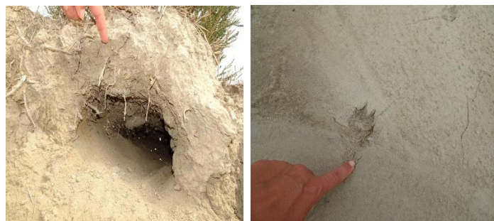
Figure 6: Nutria burrow and footprint. The animal dug the burrow in the topsoil covering the embankment, using the treated soil as bedding- September 2021 (photos S. Nicaise)
