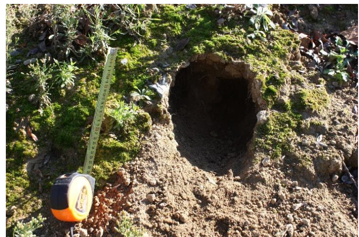
Figure 3: 17 burrows found in December 2015 on silt embankments confirm the presence of rabbits in the DigueELITE area (photos DigueELITE)
