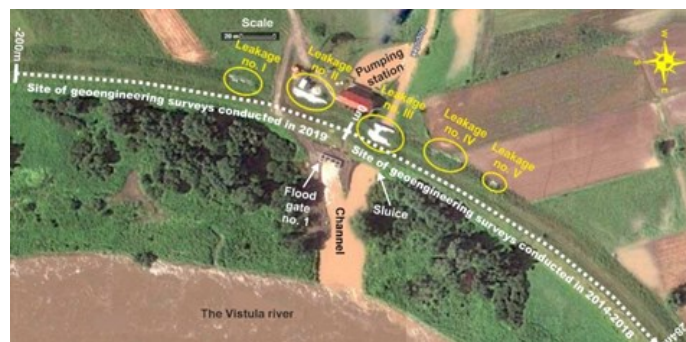
Figure 14: View of the investigated levee of the Vistula River with marking of the leakage zones observed during the great flood in 2010. (Radzicki et al., 2021)
