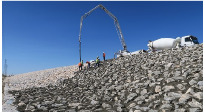
Figure 11: Levee resisting to overflow between Tarascon and Arles (left bank of the Rhône). Copyright SYMADREM.
