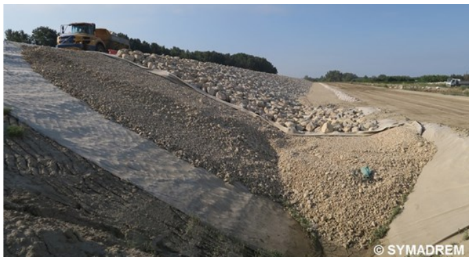
Figure 10: Cross section of the levee resisting to overflow between Beaucaire and Fourques (right bank of the Rhône)
