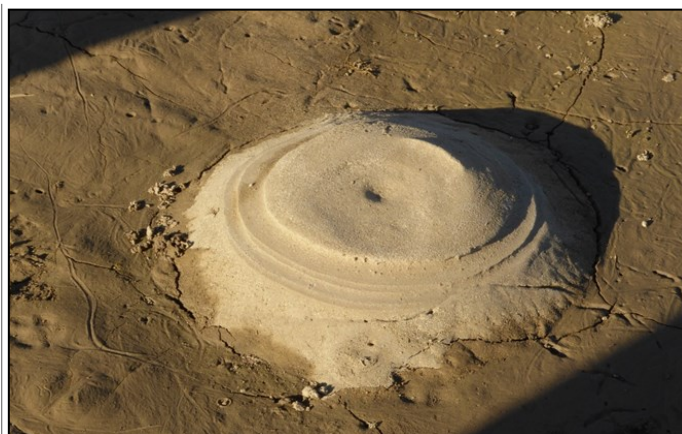
Figure 15: Sand boil near the Agly river levees (Rémy Tourment)
