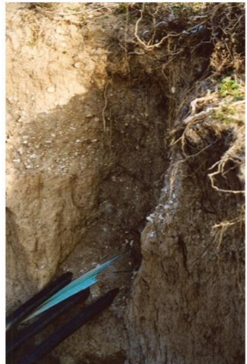
Figure set 5.5 Breach initiated along crossing cables (Mosson River, winter 2002-2003).
