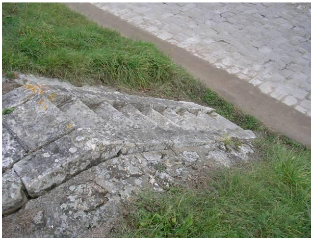
Photo 5.16 A stairway on a levee (Loire river). Transition between grass cover and stonework.
