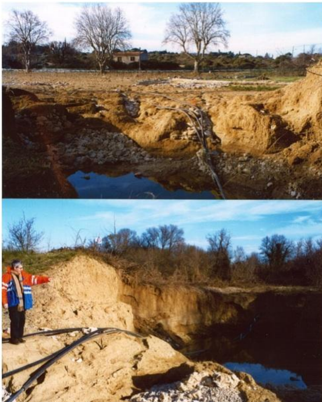
Figure set 5.5 Breach initiated along crossing cables (Mosson River, winter 2002-2003).
